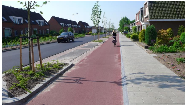
Figure 3.2.3 Separation type example on the left side of the bicycle path (Cyclenation, 2014)
