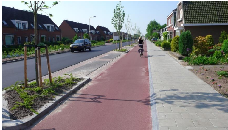
Figure 3.2.4 Bicycle path with a sloping curb as road side type (right of the bicycle path) (Cyclenation, 2014)
