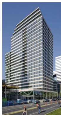
Figure 25: New Amsterdam building (VIAC, n.d.)
