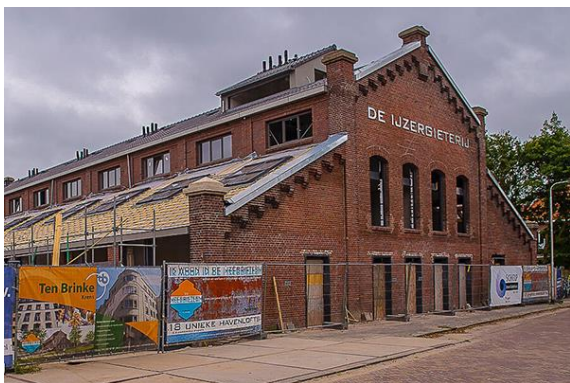
Figure 2.6. [De IJzergieterij, a former iron foundry at the Piushaven in Tilburg, built in 1900]. Adapted from Mijn Piushaven website, by F. de Roeck, 2016, retrieved from https://mijnpiushaven.nl/bouw-ijzergieterij-elf-maanden-later/ Copyright 2016 by Freddie de Roeck.
