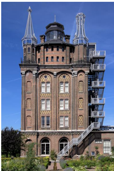
Figure 2.10. [Former water tower along the Wantij in Dordrecht, built in 1882]. Reprinted from Watertorens in Nederland website, by J. van Zegveld, 2012, retrieved from http://www.watertorensnederland.nl/watertorens/dordrecht_wantij/dordrecht_wantij.html Copyright 2012 by Johan van Zegveld.
