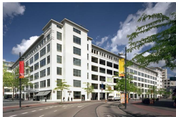
Figure 2.7. [The White Lady, a former light bulb factory in Eindhoven, built in 1926]. Reprinted from Herbestemming.nu website, by N. van Onna, 2006, retrieved from https://www.herbestemming.nu/projecten/de-witte-dame-eindhoven/ Copyright 2006 by Norbert van Onna.
