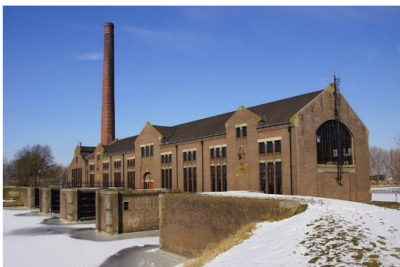
Figure 2.1. [D.F. Wouda Steam Pumping Station in Lemmer, built between 1917 and 1918]. Reprinted from Urbanplan website, by M. Reiling, 2011, retrieved from https://www.urbanplan.nl/series/woudagemaal.htm/ Copyright 2011 by Maarten Reiling.
