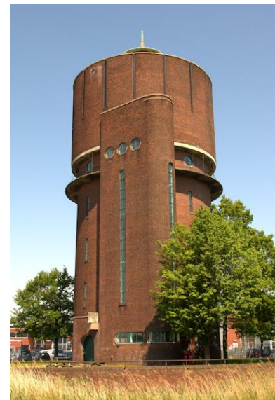
Figure 2.13. [Former Belcrum water tower in Breda, built in 1935]. Reprinted from Watertorens in Nederland website, by J. van Zegveld, 2013, retrieved from http://www.watertorensnederland.nl/watertorens/breda_speelhuislaan/breda_speelhuislaan.html/ Copyright 2013 by Johan van Zegveld.
